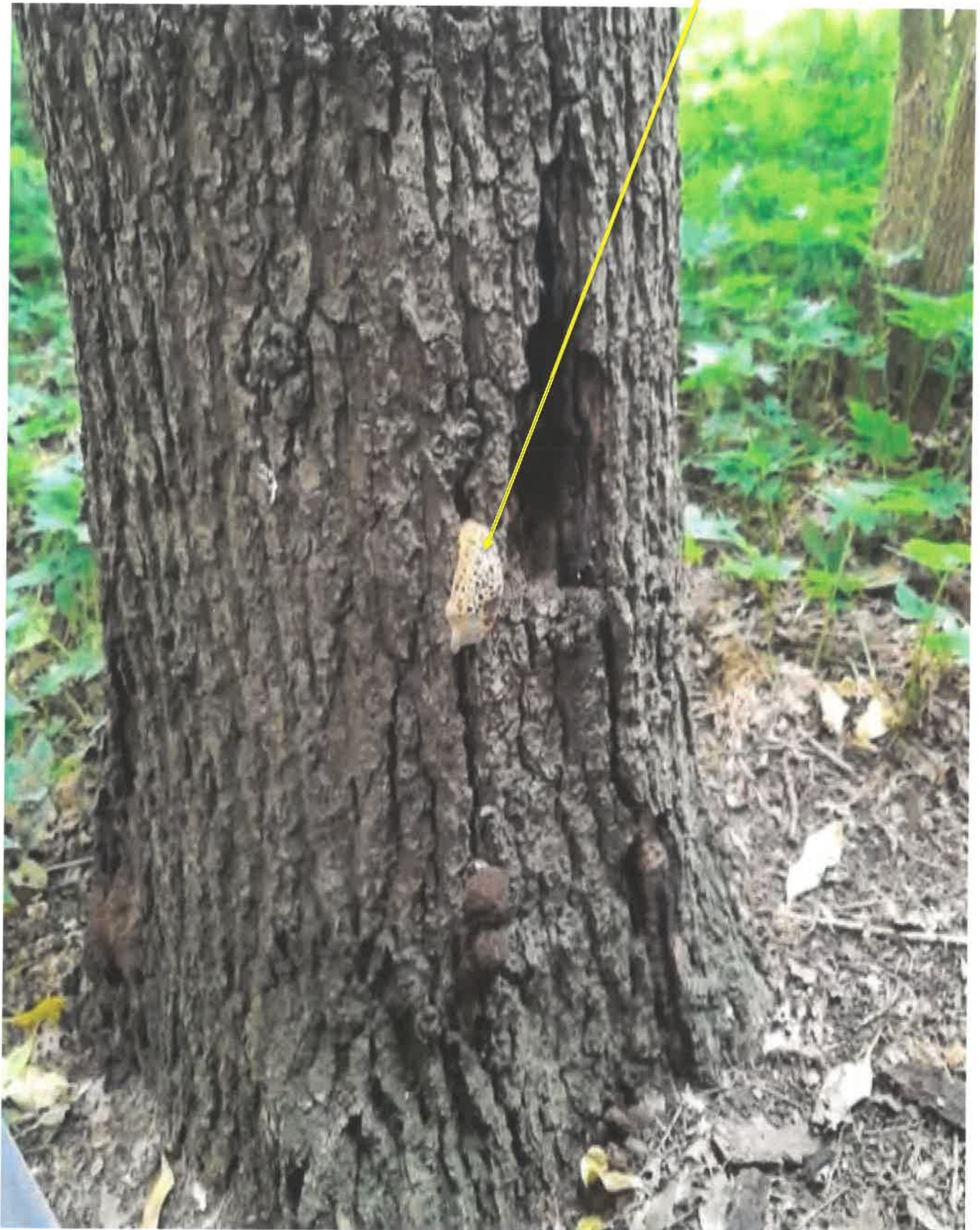
Photograph 2 – Detail of base of T1 to east, showing stem wound and Ganoderma bracket.
